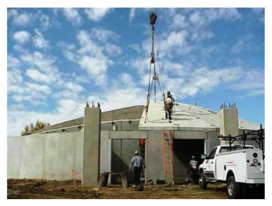
The ladder is too short to allow proper access to the work area. They are more than 6 feet above the ground and we can't tell if they are wearing fall protection but it doesn't look like it.
